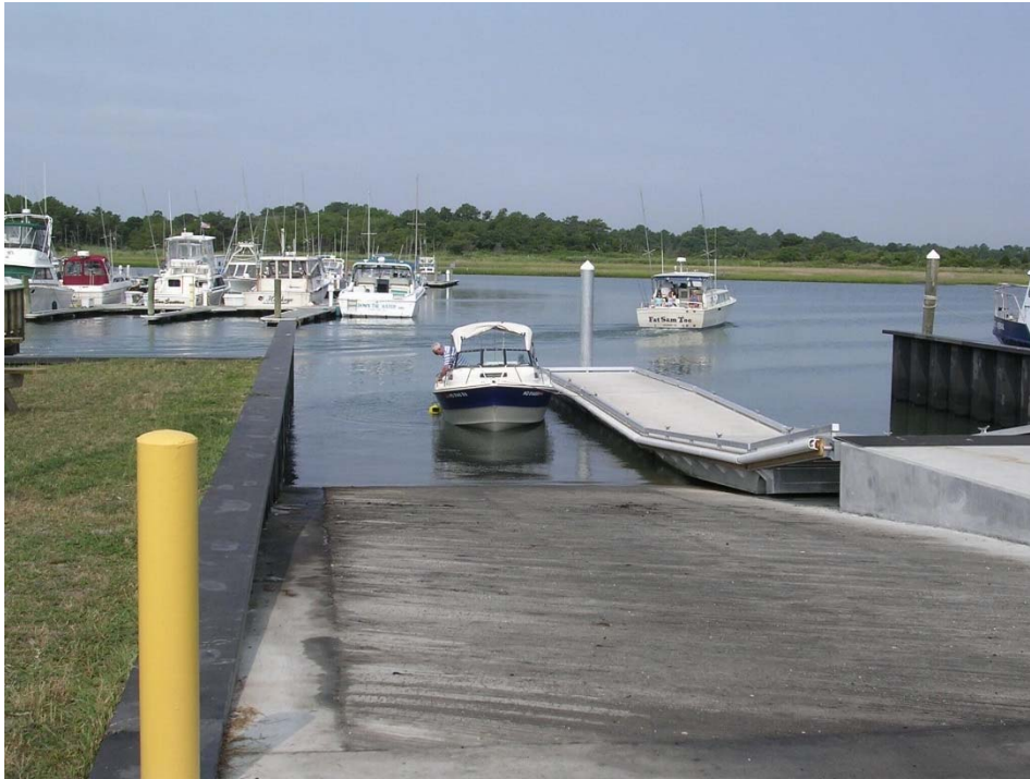
Example of Ground-Out Floating Dock
