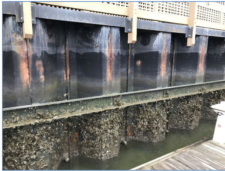
Typical Steel Bulkhead Condition at the Isle of Palms Marina
