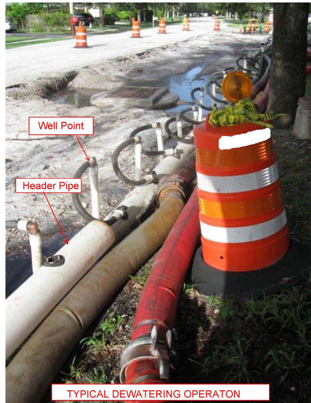
Figure A – Typical Dewatering Operation
