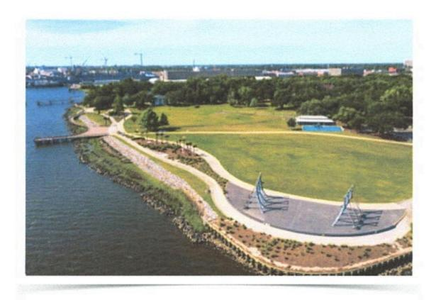
In late 2019 and early 2020, we wrapped up the Riverfront Park Boardwalk Replacement project, replacing the boardwalk and pier with composite, and adding rip-rap for erosion control.
