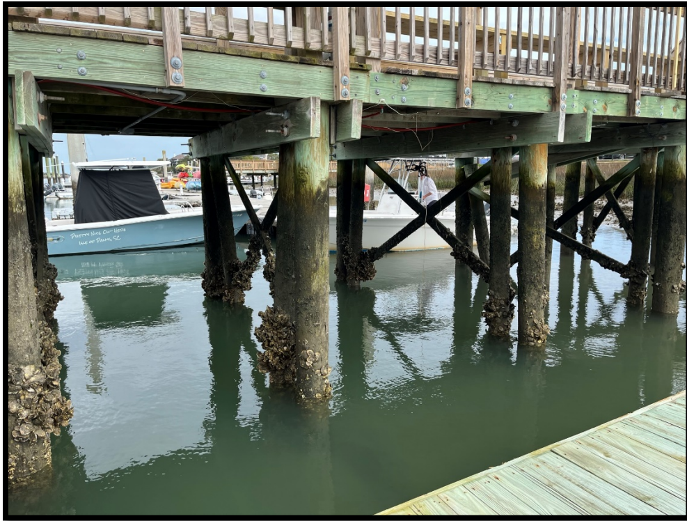
Photo 15. Timber Piles and Framing - Public Dock Access Pier
