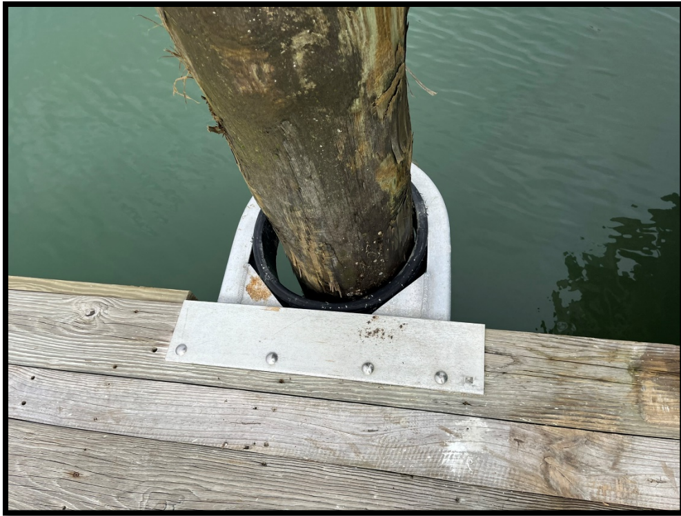
Photo 21. Anchorage Pile and Pile Guide - Public Dock
