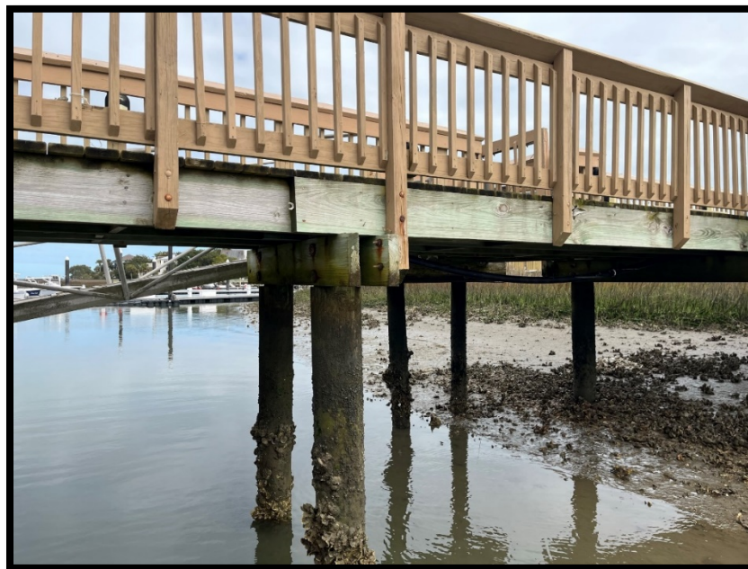
Photo 2. Timber Piles and Framing
