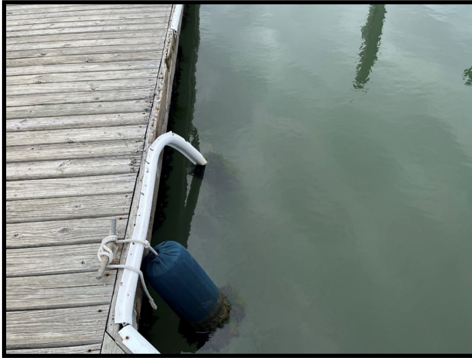
Photo 7. Timber Waler Condition and Missing Bumper Strip (Marina-Controlled Area)
