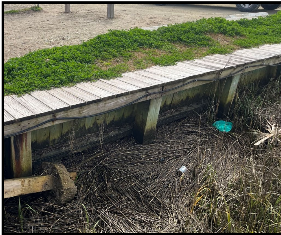
Photo 22. Timber Bulkhead Waterward Lean
