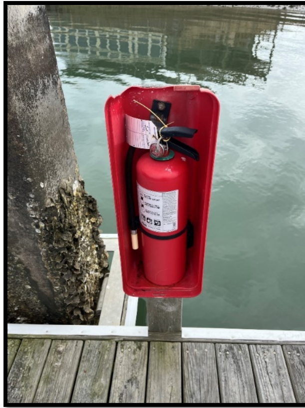
Photo 13. Fire Extinguisher with Missing Protective Covering
