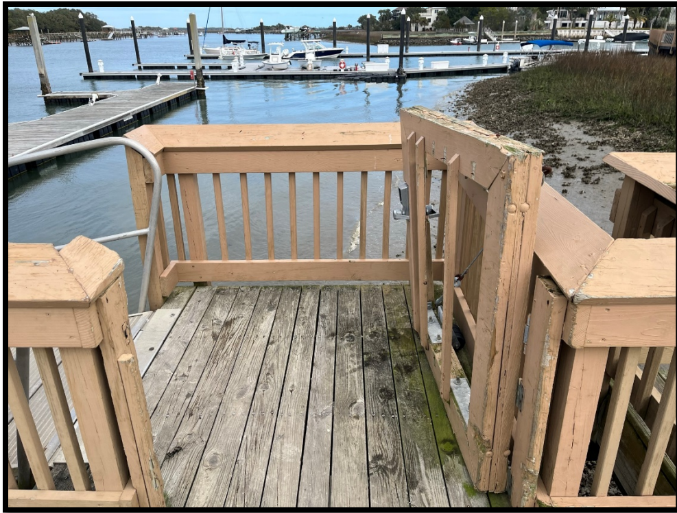
Photo 6. Damaged and Worn Access Gate
