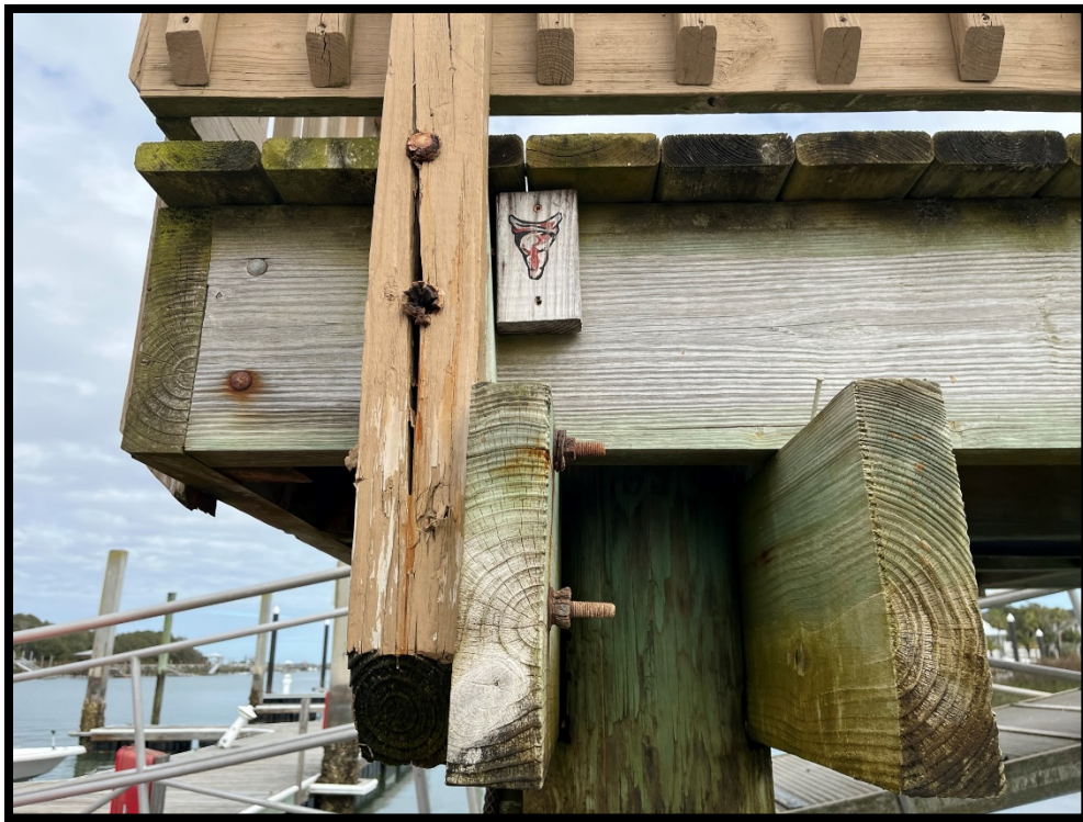
Photo 5. Cracked Railing Support
