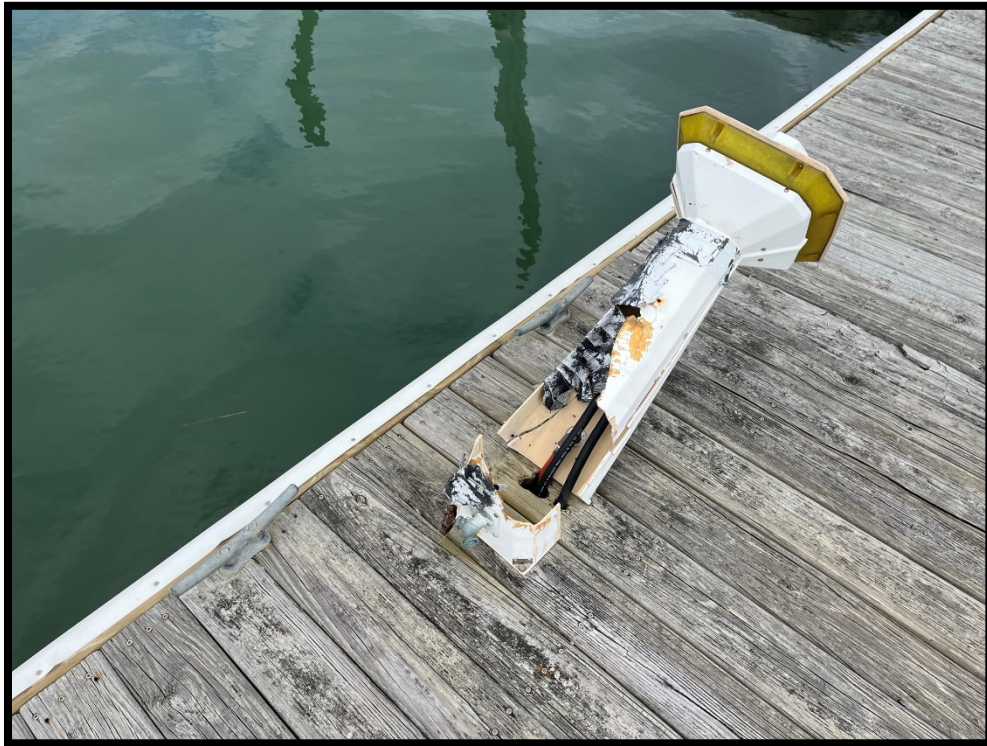
Photo 12. Utility Pedestal Damaged Beyond Repair
