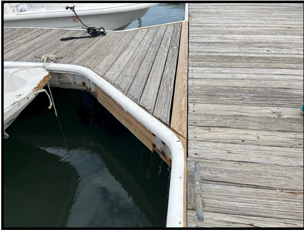
Photo 9. New Rub Rail and Select Timber Members (Restaurant-Controlled Area)
