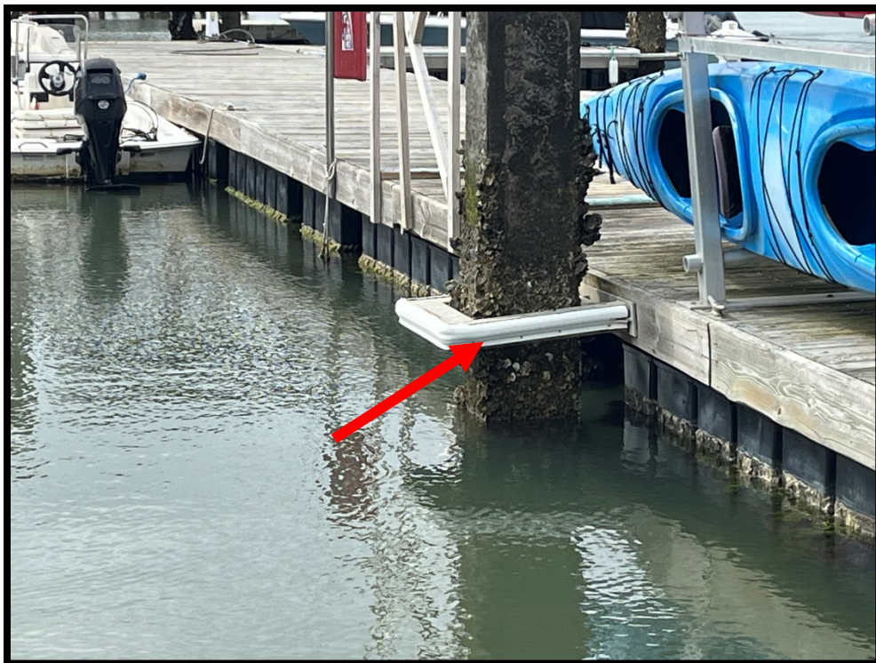
Photo 11. Loose Exterior Guide Pile
