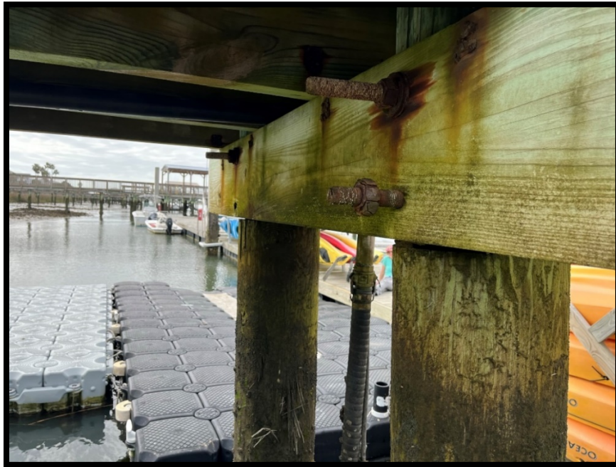
Photo 3. Severely Corroded and Missing Through-Bolts
