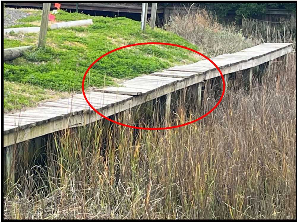
Photo 23. Timber Bulkhead with Missing Deck Boards
