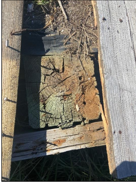
Figure 3.12. Deterioration in Top of Pile
