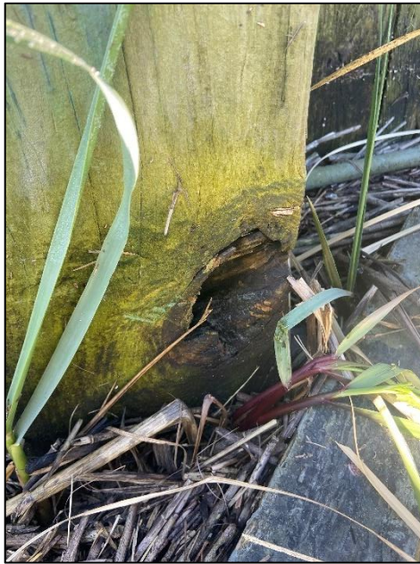
Figure 3.8. Knot in Third Pile from Pier
