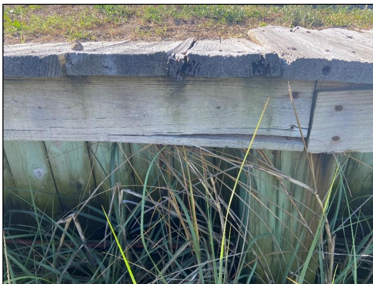
Figure 3.15. Connection with Two Rusted Nails
