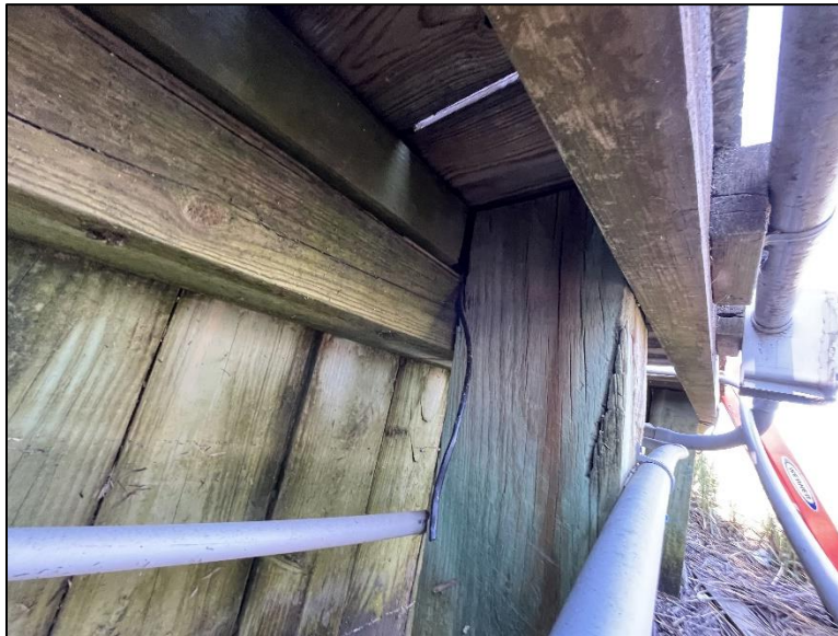
Figure 3.3. Split Top Waler Near West End of Bulkhead
