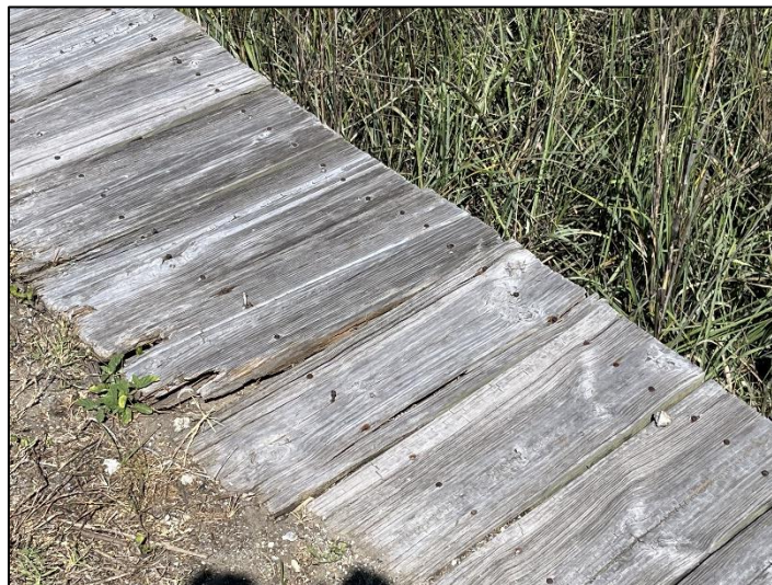
Figure 3.13. Deteriorated Decking
