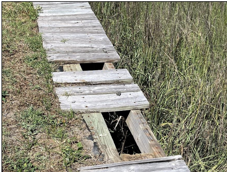
Figure 3.14. Missing Decking
