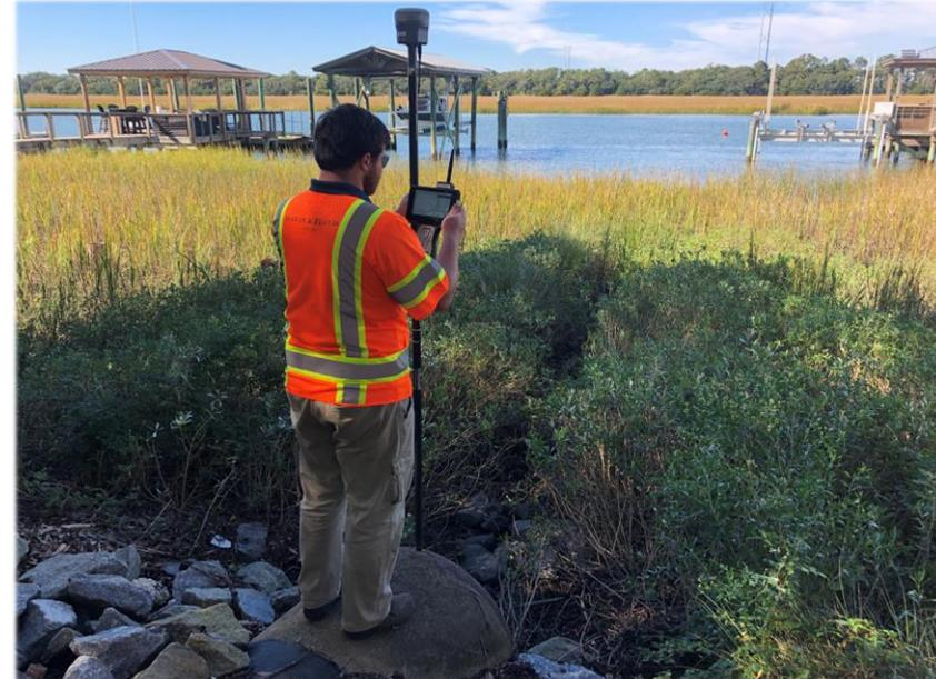
Example of surveying the drainage system inventory using the GPS units. This photo was taken at an outfall going to the intracoastal waterway.
