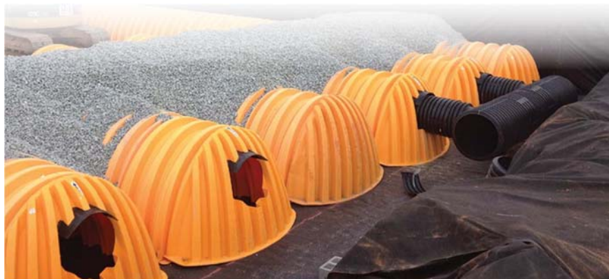
Figure 10 – Infiltration chambers being installed on a project site (photo credit to ADS StormTech).
