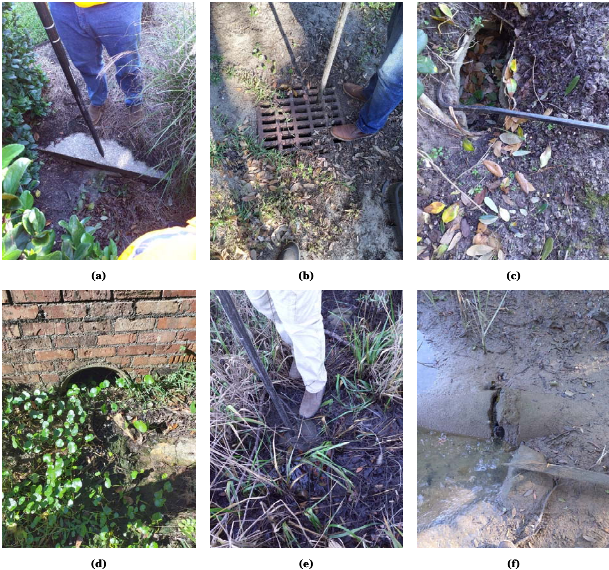
Figure 7 – Examples of visual existing conditions assessments documenting general maintenance deficiencies for: (a) silted inlet; (b) inlet with debris build up; (c) stormwater pipes which have separated; (d) stormwater pipe filled with sediment; (e) buried outfall pipe; and (f) degrading disjointed outfall pipe.
