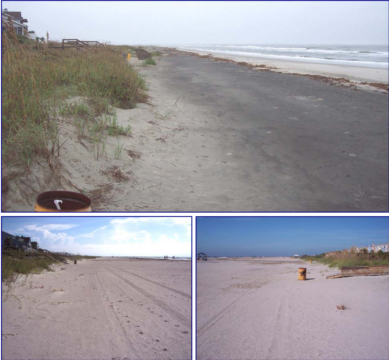
FIGURE 3.18. View northeast from station 254+00 (adjacent to Seagrove Villas) prior to the project in October 2007 (upper) and views northeast (lower left) and southwest (lower right) in September 2009. An erosional arc associated with the 2006 shoal-bypass event had formed in this area prior to the project (see Fig 3.15).
