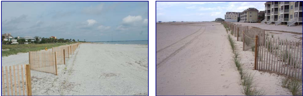
FIGURE 3.46. [LEFT] Sand fencing in the Deweese Inlet reach in May 2008, shortly after installation. [RIGHT] Sand fencing and vegetation in the North Wild Dunes reach (near Seascape Villas ) in September 2009, ~4 months after installation. Note v-shaped configuration of sand fencing, opened toward the sea, with 10 ft gaps between sections—following design guidance by SCDHEC-OCRM.
