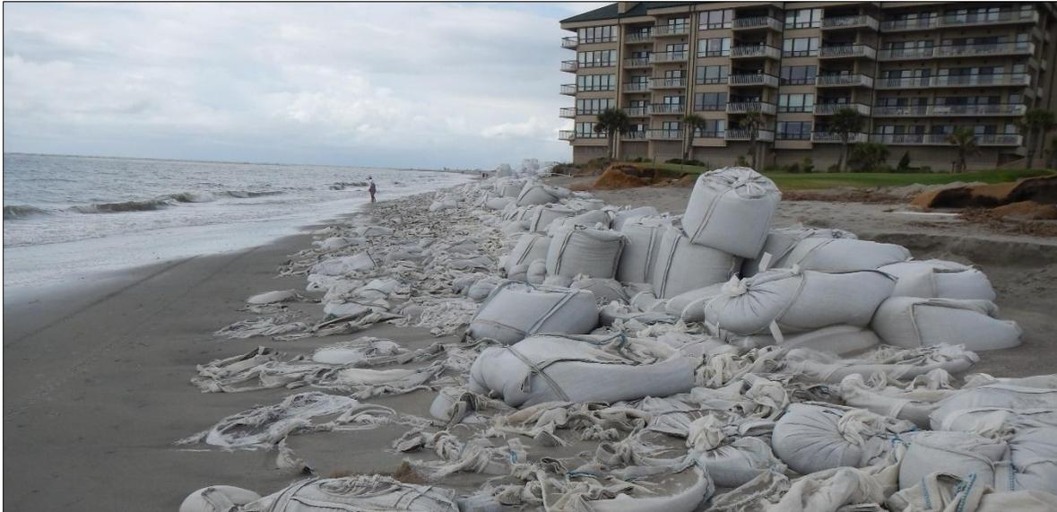
**FIGURE 2.5.** To prevent additional erosion, sandbags were installed along several structures from Shipwatch to Ocean Club from 2004 to 2007.
