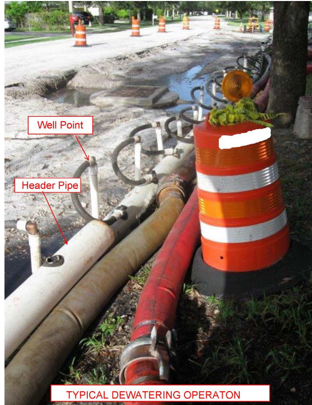
Figure A – Typical Dewatering Operation
