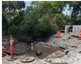
Increase storm pipe size and structure
