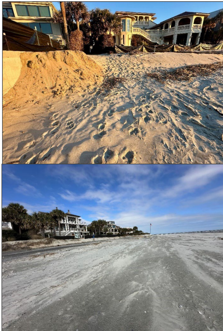
Figure 1. Photographs from recent site visit showing the high tide wrack line at the toe of the artificial dune (top photo) and a wide flat beach lacking a dune (bottom photo).
