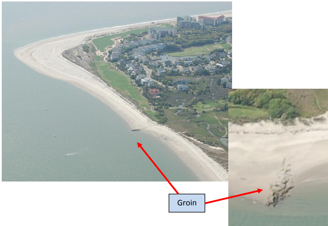
Figure 20. April 14, 2011 photos of groin at Wild Dunes Links Course, 17 th tee.
