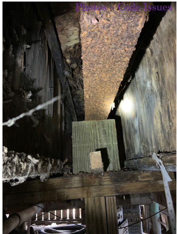
Steel beam blocked up, no connectivity
