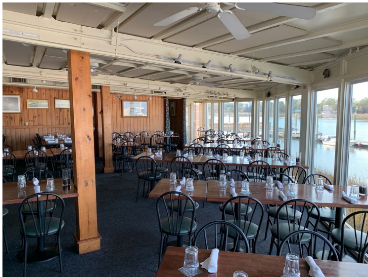
Infill porch slopes approximately 6 inches, creating a significant cross-slope in the room.
