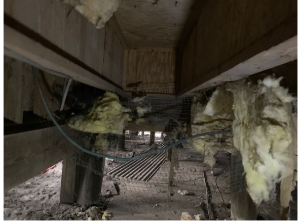
Pile foundation. Insulation falling down
