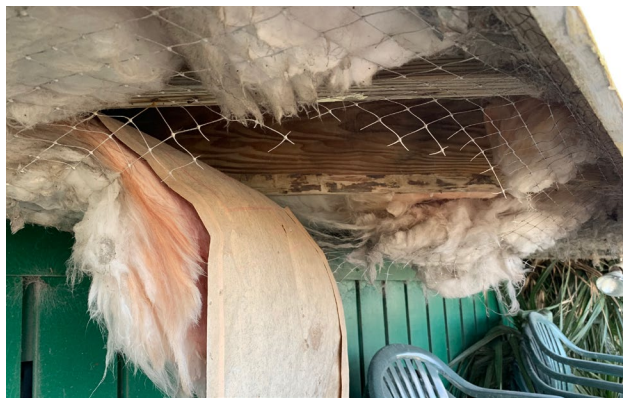
Insulation falling down or missing in floor
