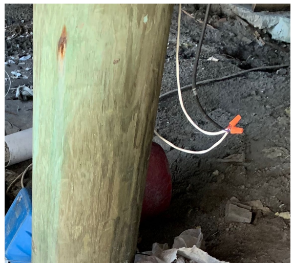
Open electrical connections
