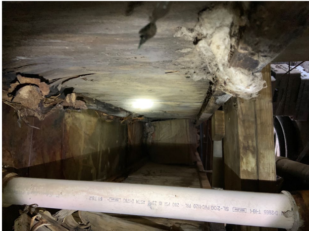
Plywood totally deteriorated. Underside of cooler.
