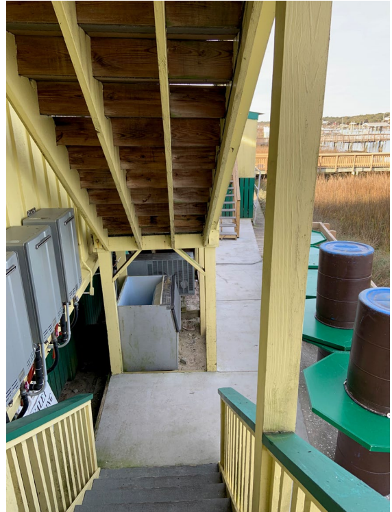
Egress, railing discontinuous Lack of egress lighting
