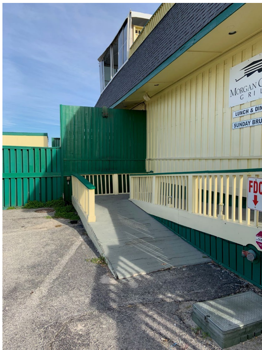
Start of ramp to first floor. Note electrical box in the way of the landing and the railing ending before the bottom of the ramp.
