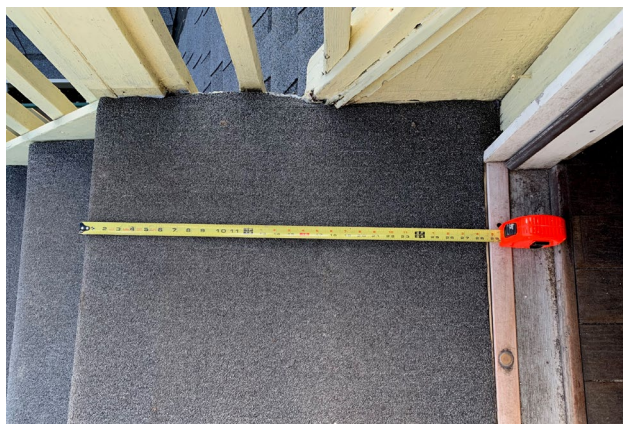
Insufficient landing depth at top of stair
