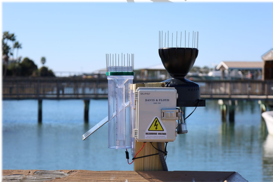
b) Example Monitoring Station
