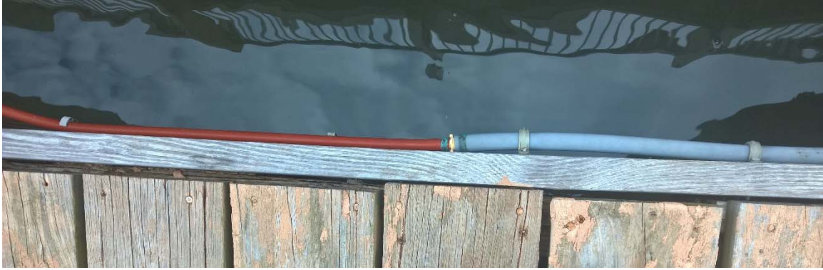
Different Types of Piping and Different Sizes Connected (Lack of In-Dock Conduit Space)
