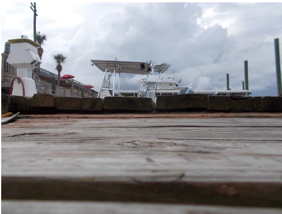
Uneven Deck/Framing Failure at Existing Fuel Dock
