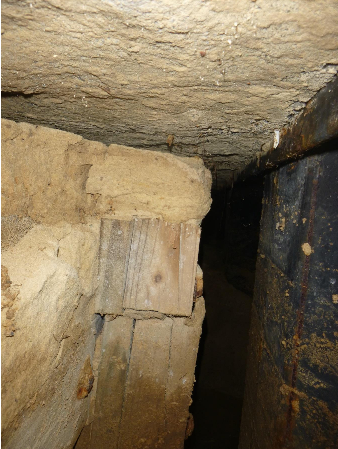
Photo 1: Void between walls
