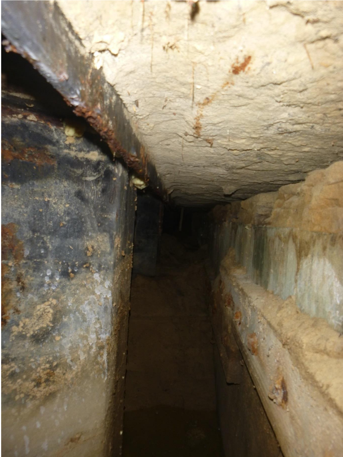
Photo: Void between walls
