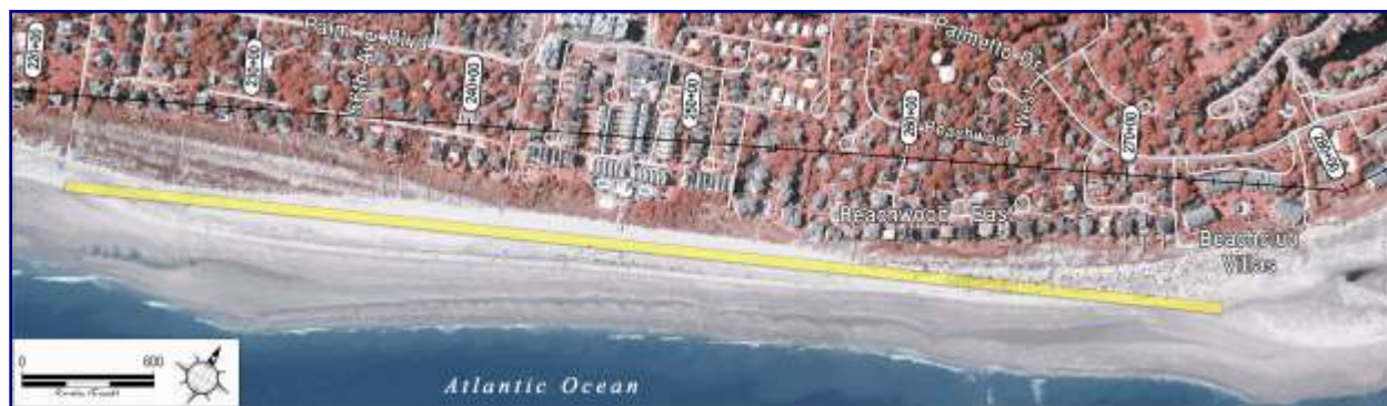
FIGURE 3.13. Reach 5 spans from 53 rd Avenue (station 222+00) to the Wild Dunes POBH (station 280+00). The approximate limits of nourishment Reach A are identified by the green bar. [March 2009 aerial image by Independent Mapping Consultants Inc]
