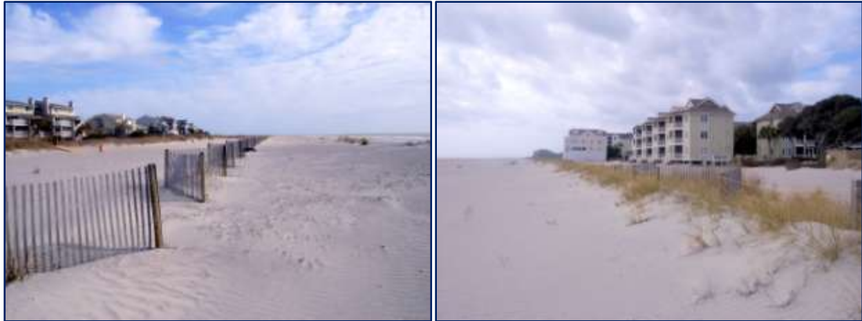
FIGURE 3.50. [LEFT] Sand fencing in Reach 5 in February 2011. Less sand has accumulated in this area than in Reach 6. [RIGHT] Sand fencing and vegetation in Reach 6 (near Port O Call) in February 2011, ~22 months after installation. Over 2 ft of sand has accumulated in a generally continuous dune.
